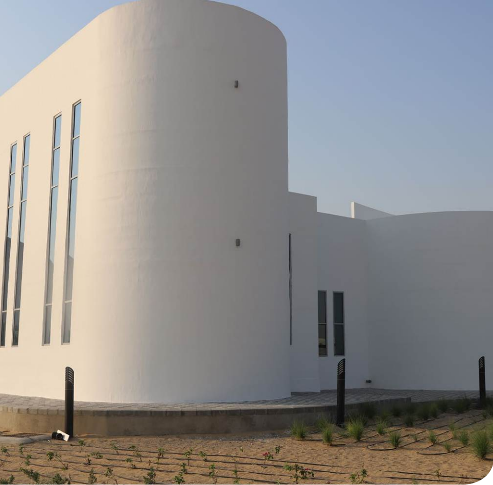
At 31 feet tall and more than 640 square feet in area, the government building in Dubai is the largest 3D-printed building to date. Courtesy of Apis Cor.
