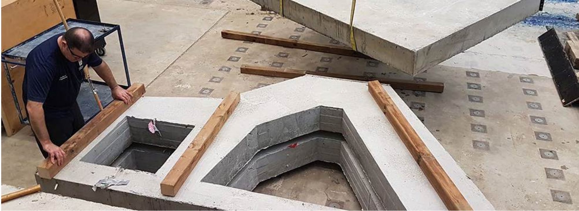
A concrete deep beam created through generative design. Courtesy of Dr. Sreekanta Das's Research Group.
