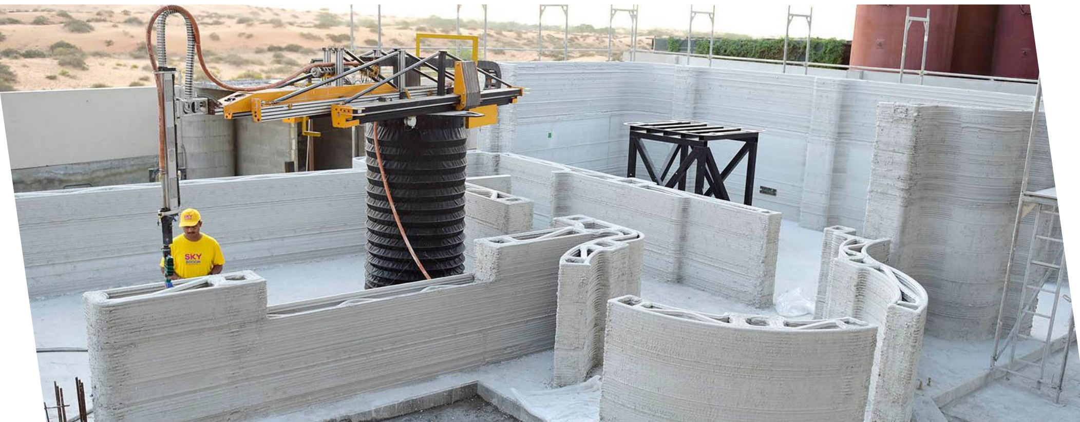
A 3D-printed structure takes shape. Courtesy of Apis Cor.
