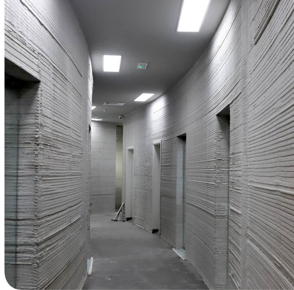
Internal walls made using a 3D-printing process. Courtesy of Apis Cor.
